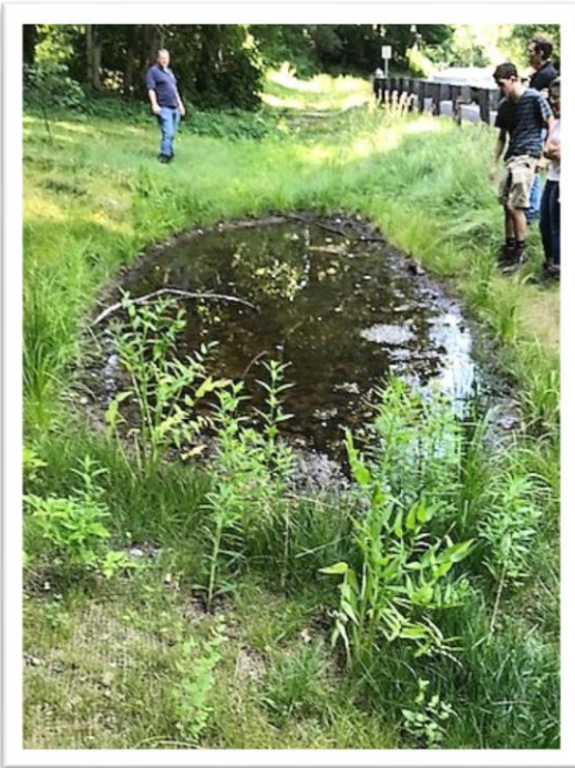
At the Inwood tributary, runoff from the Inwood neighborhood is diverted by a large Ash tree log into an infiltration area shown in the background of the picture below. The infiltration area is a depression in the ground where the rain water collects and soaks into the soil (good soil percolation). Large Ash tree branches were added to the depression to help create habitat for a healthy ephemeral pond. During the fall, winter and spring, water is present in the depression, thus creating an ephemeral pond. By creating
